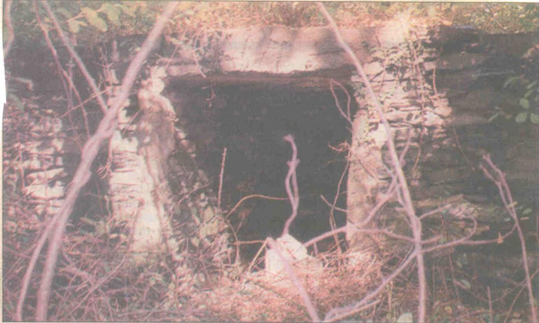
Above, the crypt at the Hill/Allen family cemetery in Quidnessett dates to the late 1700s. It is entirely constructed of field stones and is missing its cast iron door. Below, the Elm Grove crypt was constructed in the mid-1800s and could hold a number of coffins awaiting the spring thaw.
